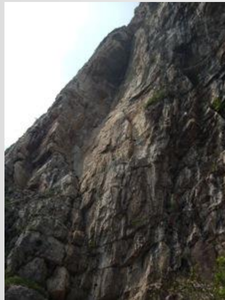
The monitored mountain wall
